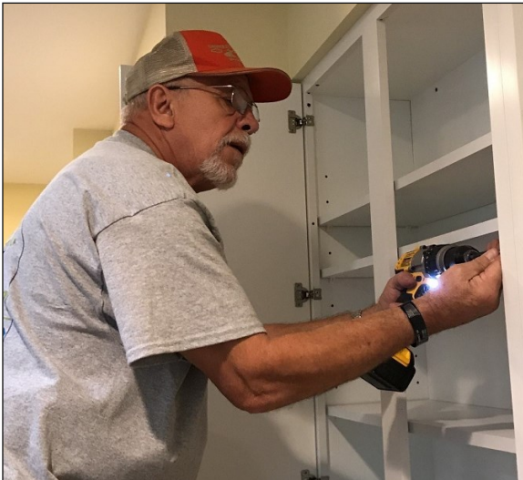
Volunteer Robin Holycross deconstructs kitchen cabinets to sell in the ReStore.
